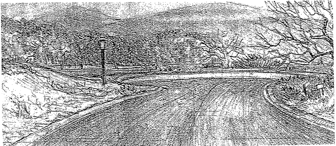
Cul-De-Sac with Proper Road Width and Turnaround
